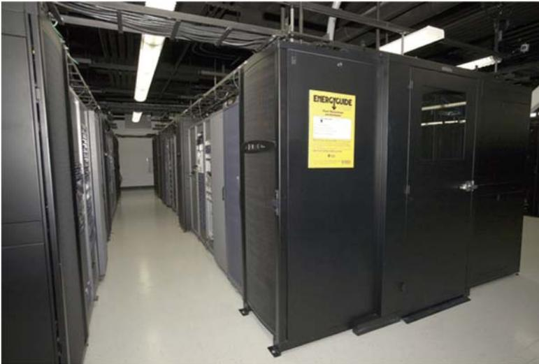
Figure 5. The use of hot aisle containment with in-row cooling makes pods self-sufficient from a cooling perspective.
