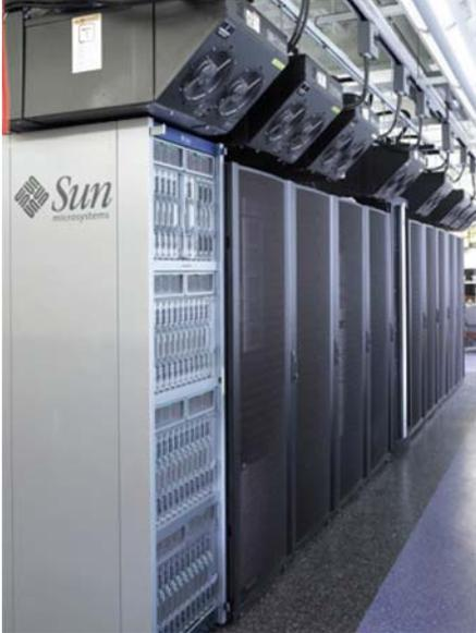
Figure 6. Overhead cooling units can effectively cool high-density racks in raised floor or slab configurations.
